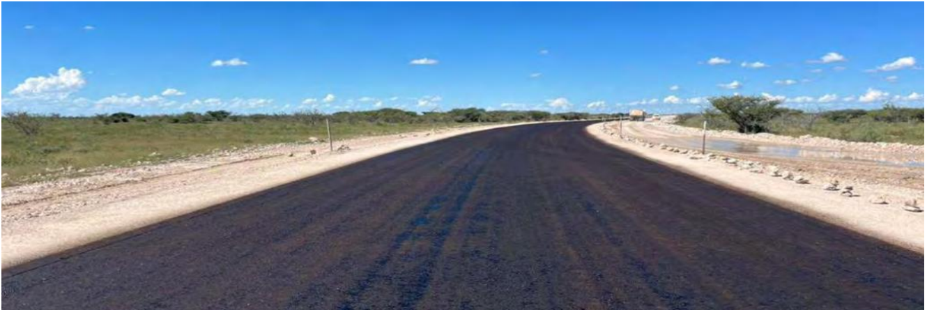
Photo 1: Section 1: 0-20km Okaukuejo – Halali: Bitumen Primed section (approx. km 0+560)
