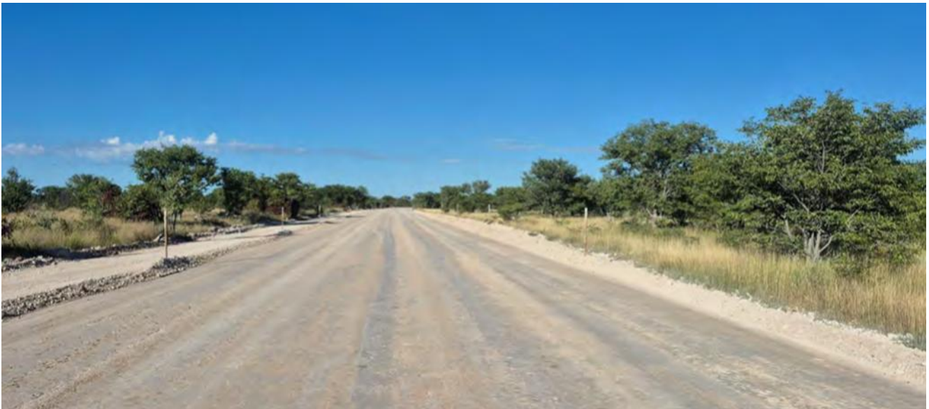
Photo 2: Section 1: 20-40 km Okaukuejo-Halali: Completed Roadbed (Final Fill) layer (approx..km28+920)
